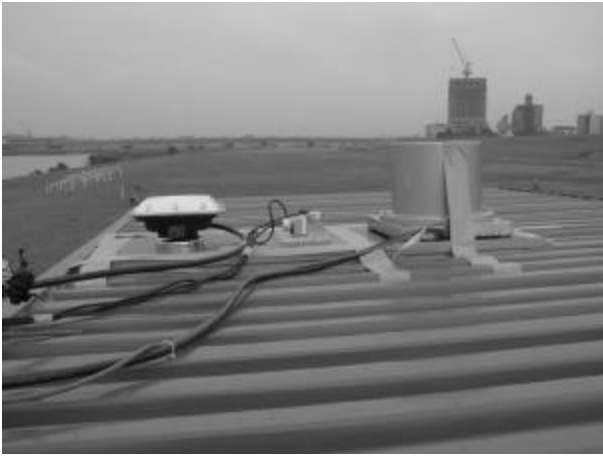
Figure 2. The setup of GPS antenna, accelerometer, and velocimeter.
