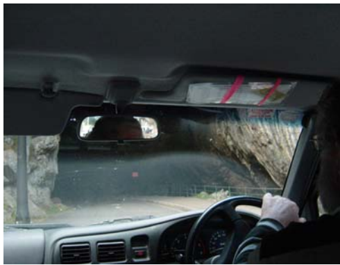
(a) Entrance of the tunnel
