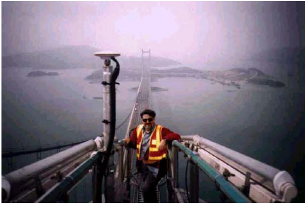
Fig. 6 GPS antenna on Tsing Ma Bridge, Hong Kong. The bridge has over 800 sensors of which 31 are GPS. The GPS sensors continuously monitor motion caused by high winds and traffic.
