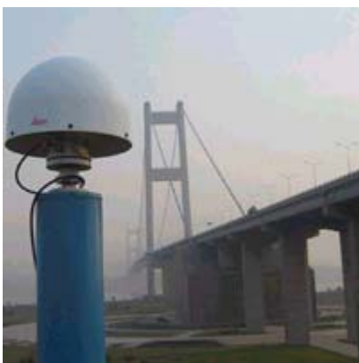
Fig. 8 GPS monitoring station at Jiangyin Bridge, China.
