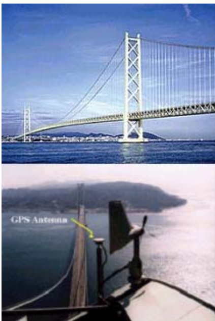
Fig. 7 Akashi-Kaikyo Bridge, Japan. In the bottom image is a GPS antenna on one of the bridge towers.
